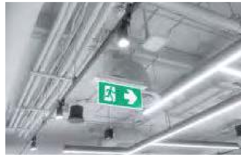
Mechanical, Electrical & Plumbing (MEP)
